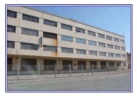
**Site Description:** A large, 262-by-262-foot, four-story reinforced concrete, flat-roofed warehouse that includes banks of industrial steel sash in horizontal bands across all four stories, except at the front (south) of the first floor. The front has a bank of steel roll-up industrial doors extending the length of the concrete loading dock area. The loading dock is sheltered by a concrete canopy (HRA-1118, pp 70-71). Figure 8.3.4.18 provides a map of the site location.
